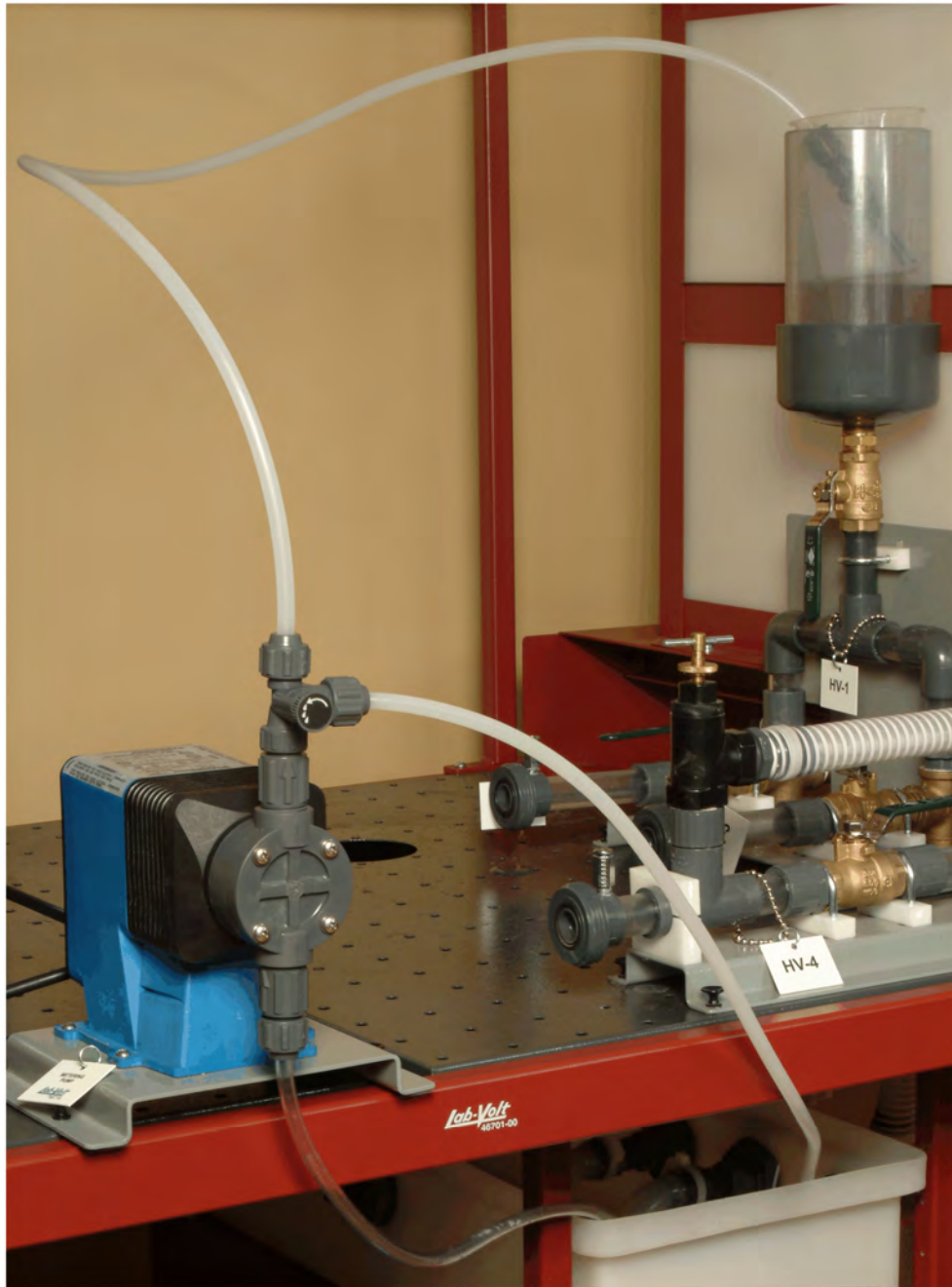
Figure 1-5. Installation of the Metering Pump on the Pump Bench.
